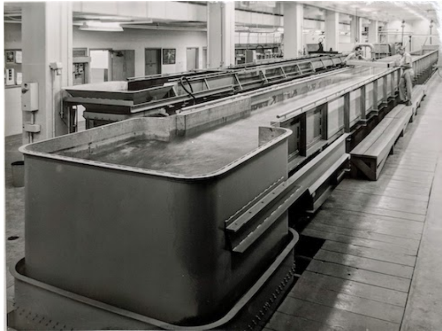
The newly built 40-meter flume in the Keck Hydraulics Lab. Caltech Archives Photo
