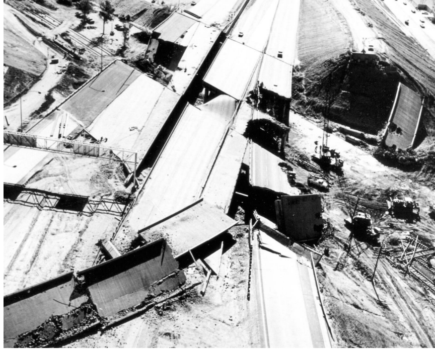
Aerial view of collapsed highway overpasses and bridges at the interchange of the Foothill and Golden State Freeways after the 1971 San Fernando earthquake. USGS Photo
